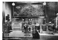
170 kW transferred 175 km from Lauffen hydropower station to the exhibition area at 13000-14700 V
